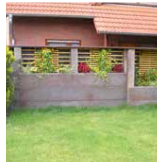
Partition wall with plants
