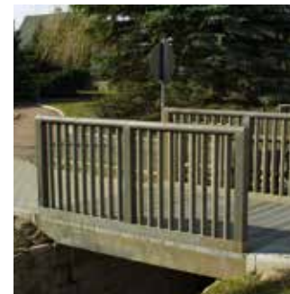
Bridge with railings and decking
