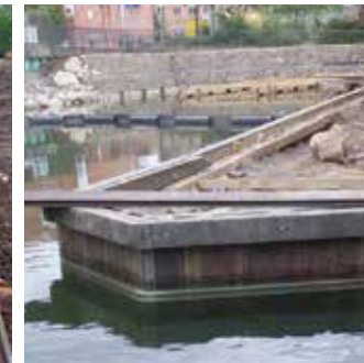
Sheet piling port with rubbing strips
