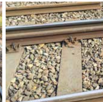
Trackbed of tram line in Berlin
