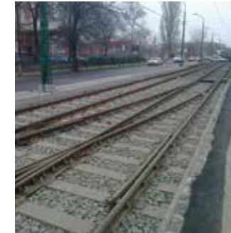
Railway switch in Budapest (Tram)
