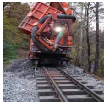
Filling of trackbed
