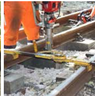
Screwing the rail on the railway tie
