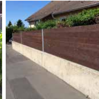
Visual and noise barrier
