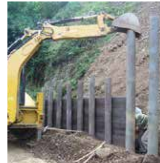
Foundation for protective wall
