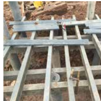
Pile substructure for viewing platform
