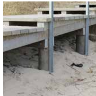
Staircase design and construction stages for beach access
